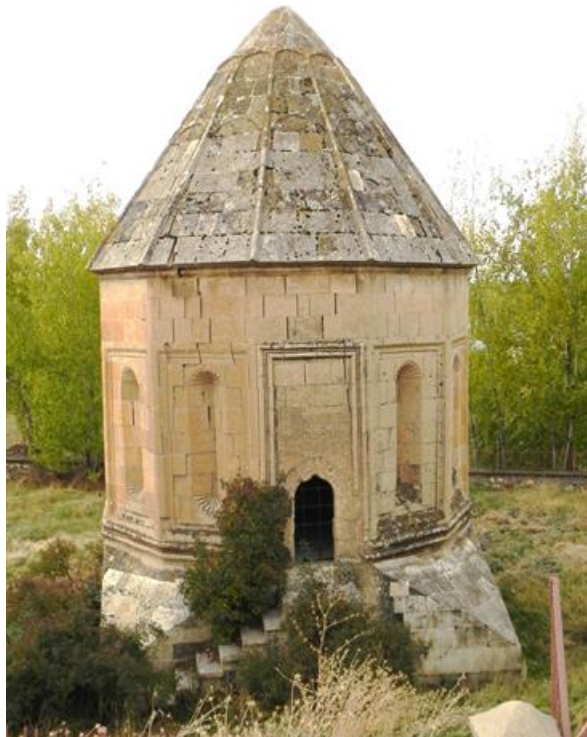
Figure 11. General view of tomb of Kadem Paşa Hatun and bed-sliding damage
