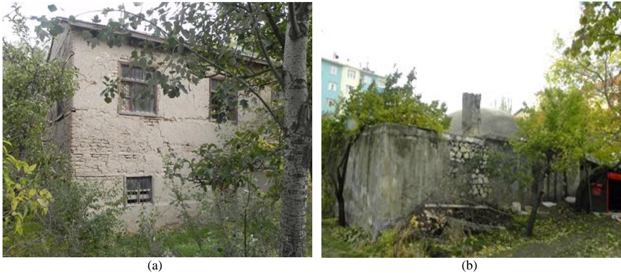
Figure 9. Mud-brick masonry building and the hammam in the same yard
