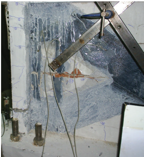
Figure 13 Damage state of specimen SA1.7-CVs at 0.86% drift level.
