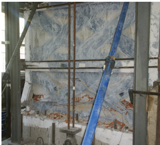
Figure 15 Damage state of specimen SA2.3-CCM at the end of loading scheme.
