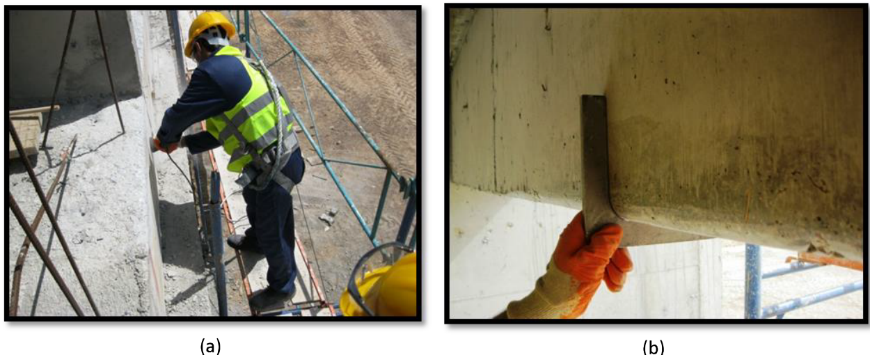
Figure 2: Concrete surface preparation and corner rounding proses
